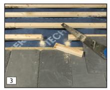
Use the trimmed slates to mark a 270mm long gap in the middle batten. Cut out this section of batten
