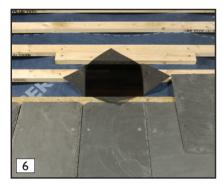
Cut the underlay diagonally and pin back onto the surrounding battens and rafters. For rigid sarking board, cut-out the rectangle.
