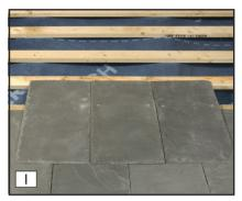
Decide in which course the vent is to be fitted and lay slates up to the course below. Lay the two slates directly below the vent.
