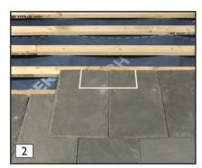
Mark the area of the two slates to be removed (hatched area shown above). Cut out this area.
