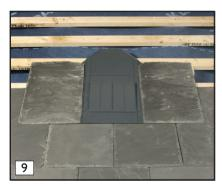
When fixing the adjacent  $400 \text{mm} \times 250 \text{mm}$  slates, they should abut the main vent body (see guide marks on vent).
