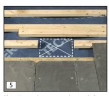
Using the cut slates as a template, mark the underlay diagonally as shown. This is the cut-line
