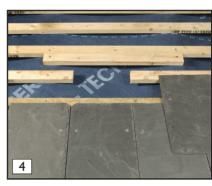
Fix an additional 1.2m support batten above the cut batten (spanning two rafters) and nail to the adjacent rafters.
