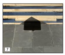
Fix the cut slates in position, leaving the underlay opening exposed.
